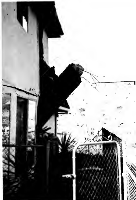
Photo 8. Damaged reinforced brick chimney in heavily damaged new district near Pacoima Dam.
